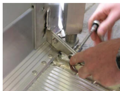
3. Assembly of side parts: - with 7 screws 10 x 60 + nuts; each rail 2 pieces to upper drill-holes; Exception: side with remote control pedal , this side up only 1 screw - and 3 screws 10 x 80 + nuts; each rail 1 piece to lowest drill-hole; Exception: side with remote control opening no screw at bottom
