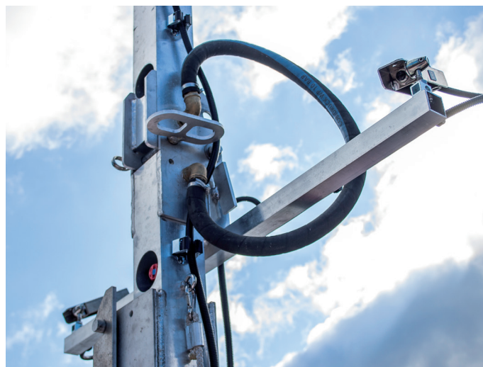
Storm nozzles and passage control
