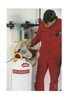
Do not enter the compartment during or 2 hours after disinfection process. Rinse pump thoroughly with water after disinfection.
