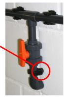
For mounting to ceiling: fixate suspension hooks with Spax screws to ceiling.
